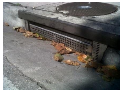
Trash excluder - this keeps trash from entering the stormwater system and can be used in conjunction with connector pipe screens.
