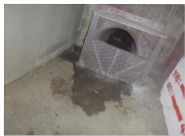
Connector pipe screen - this device captures trash after it has entered the storm drain while allowing water to flow through.
